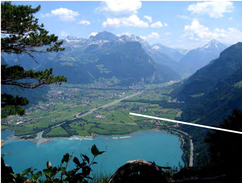
Urner Reussebene at Flüelen-Amsteg
